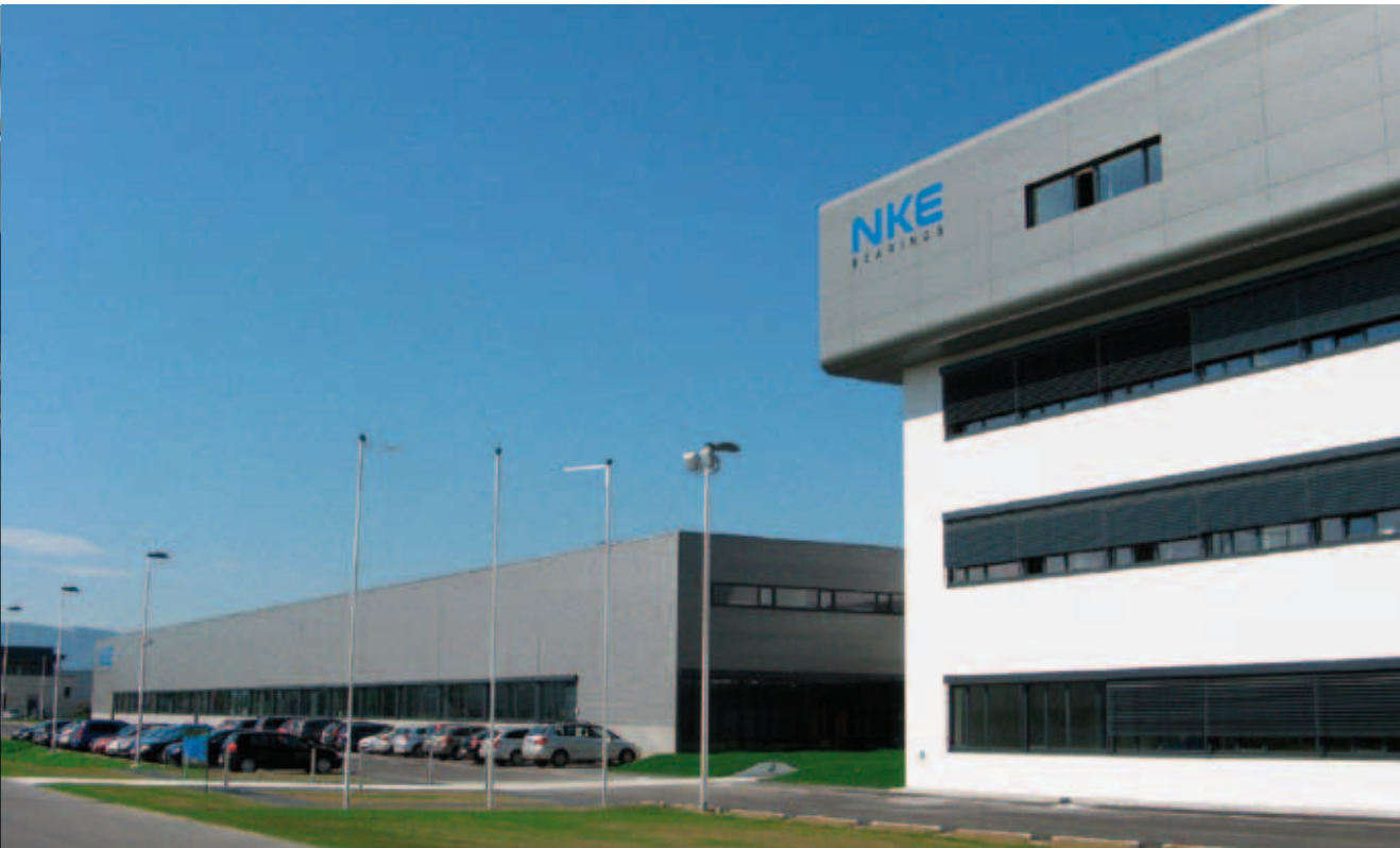
The NKE headquarters in Steyr, Austria
